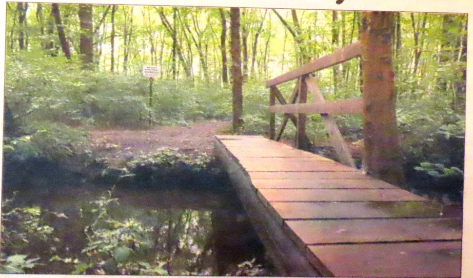
Picturesque Brotherton Bridge spans the Allendale Brook at the Celery Farm.
